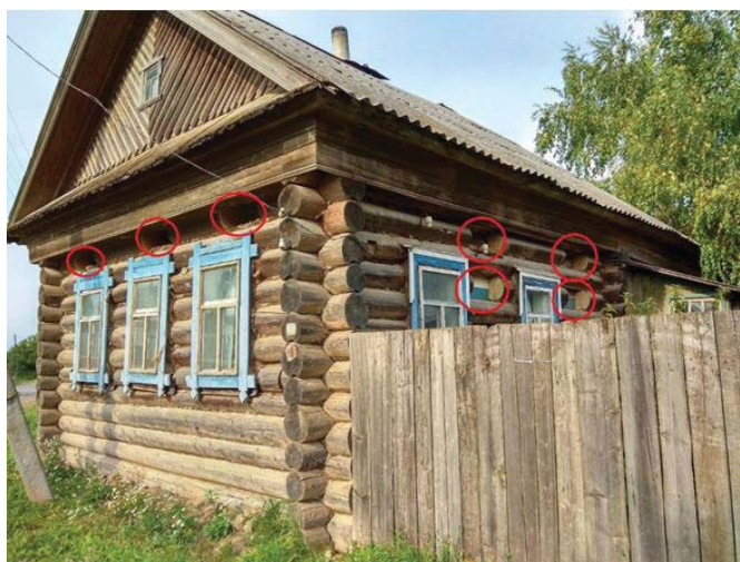
Figure 1: Facade wall (3 windows) and southern wall (2 windows) of the object of study (ovals mark the places for selecting shock bolt-fragments from the house)
